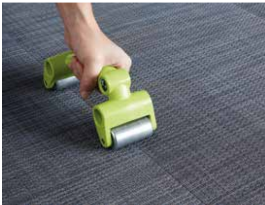
Smooth down the joints using the small seam roller.
