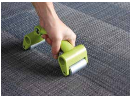
Smooth down the joints using the small seam roller.
