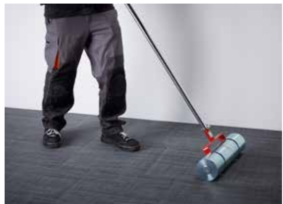
Smooth down the entire flooring area using the large, heavy roller.
