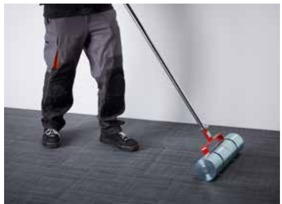
Smooth down the entire flooring area using the large, heavy roller.
