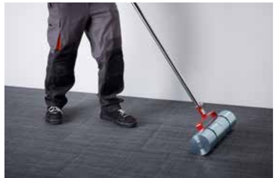
Smooth down the entire flooring area using the large, heavy roller.
