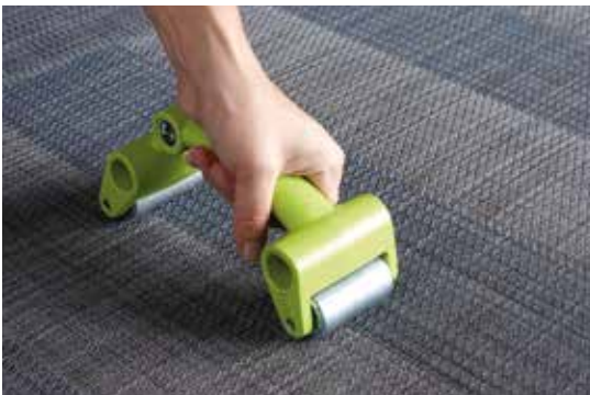
Smooth down the joints using the small seam roller.
